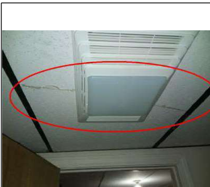
Basement bathroom ceiling
