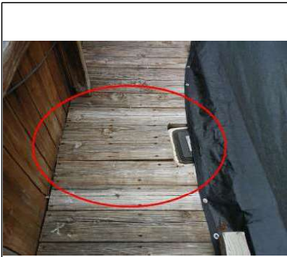
Loose boards at deck
