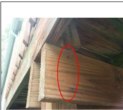
Loose boards at deck
