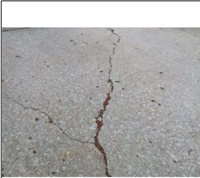
Driveway cracks
